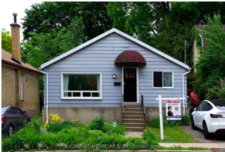
Figure 1: North Facade of the house facing Water Street. Large window to be enlarged and replaced, door to be replaced, and small window beside door to be replaced.
